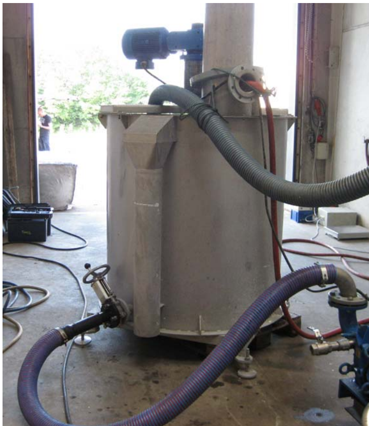
Figure 3 Stirred tank for biomass addition in test
