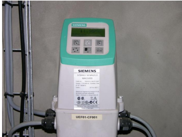
Figure 3. Flowmeter measuring amount of treated biomass.
