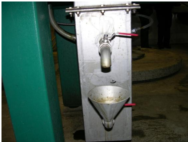
Figure 5. Tap for taking samples of liquid output.
