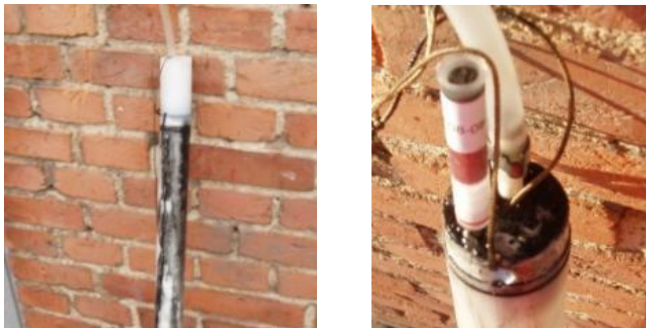
Figure 13 Pictures of Sorbisense equipment retrieved from well C14 at Søbørg Hovedgade.
