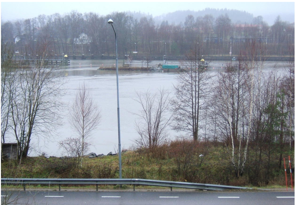
Figure 2-1 View of the river Göta älv from the premises of Lilla Edet water works.
