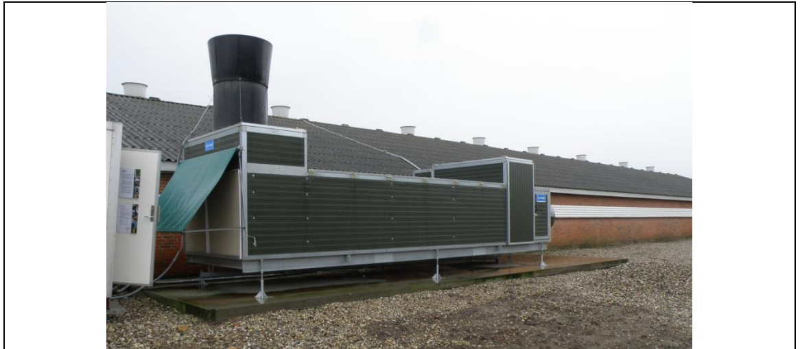
Figure 2. Picture of the Agro Clima Unit situated outside a broiler house. Ventilation air to and from the broiler house are drawn through the Agro Clima Unit by a countercurrent principle to utilise the heat content of ventilation air to heat up inflowing air.
