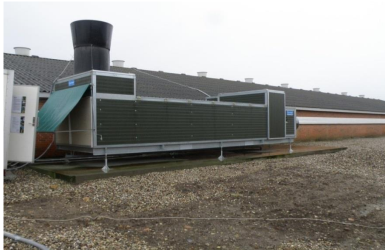
Figure 1. Picture of the Agro Clima Unit situated outside a poultry house. Ventilation air to and from the poultry house are drawn through the Agro Clima Unit by a counter current principle to utilise the heat content of out flowing air to heat up inflowing air.
